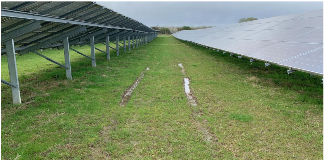
Photo 49: Ruts Caused by Vehicles
