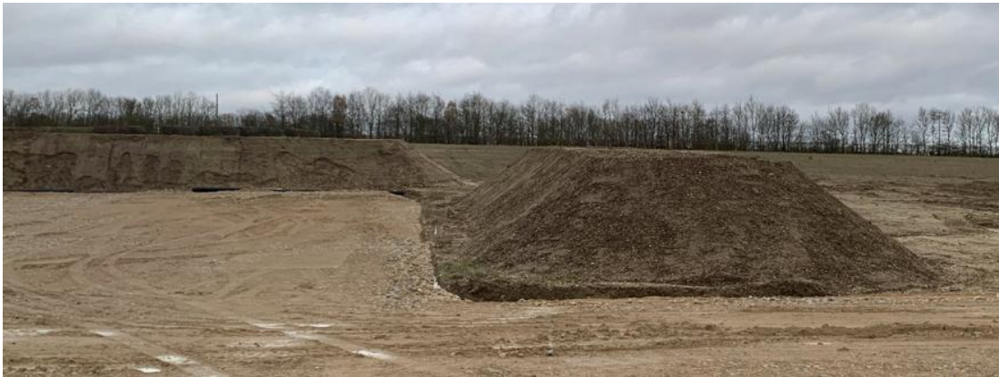
Photo 35: Topsoil Storage Example
