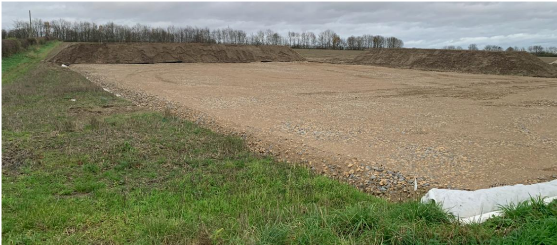
Photo 33: Newly-laid Construction Compound (Elsham-Lincoln Pipeline)
