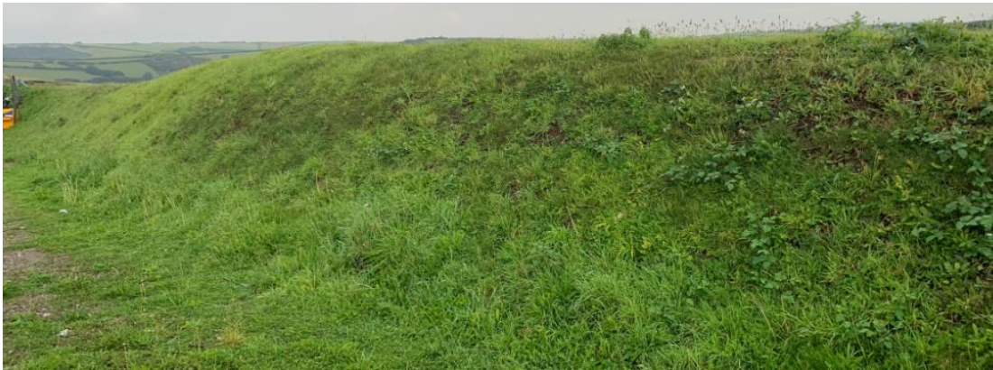
Photo 36: Grass-seeded Soil Storage
