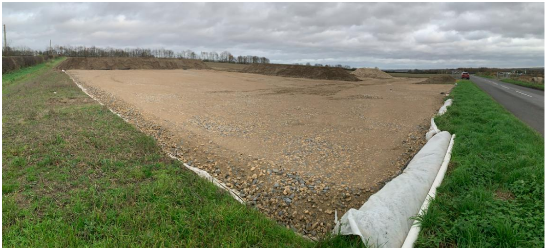
Photo 44: Example of a temporary construction compound
